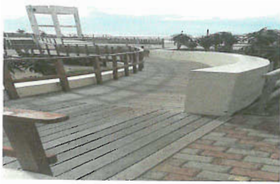
The top landing area leading to the toilet facilities.
